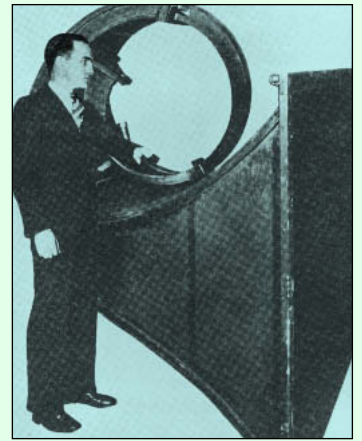
Fig. 3. Western Electric "Roxy" horn type 12A with 555W dynamic driver. (Photo, Cowan, p. 329.)
