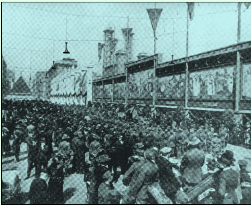
Fig. 1. First use of a distributed sound system, New York, Park Avenue (1919). Note trumpet horns in upper left hung above crowd aiming downward. (Photo from Lester Cowan Recording Sound for Motion Pictures , McGraw Hill, New York, 1931.)
